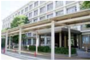
Main Research Building
