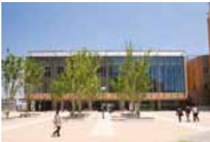
Ito Library (completed in 2009)
