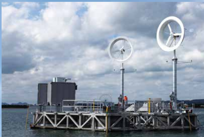
Power system experiment using Wind Lens turbines mounted on a floating platform in Hakata Bay
